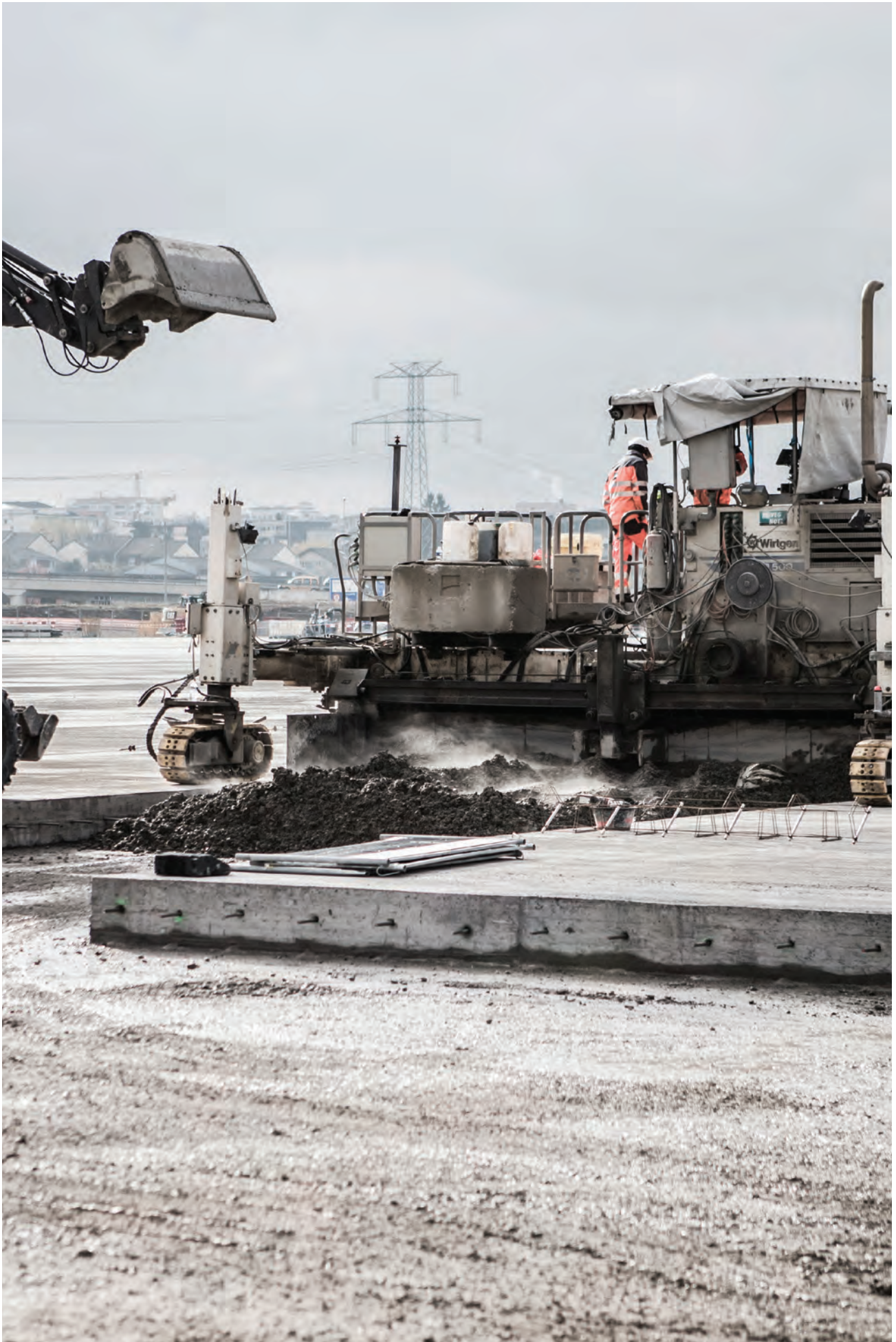
Work on the P48 parking site
