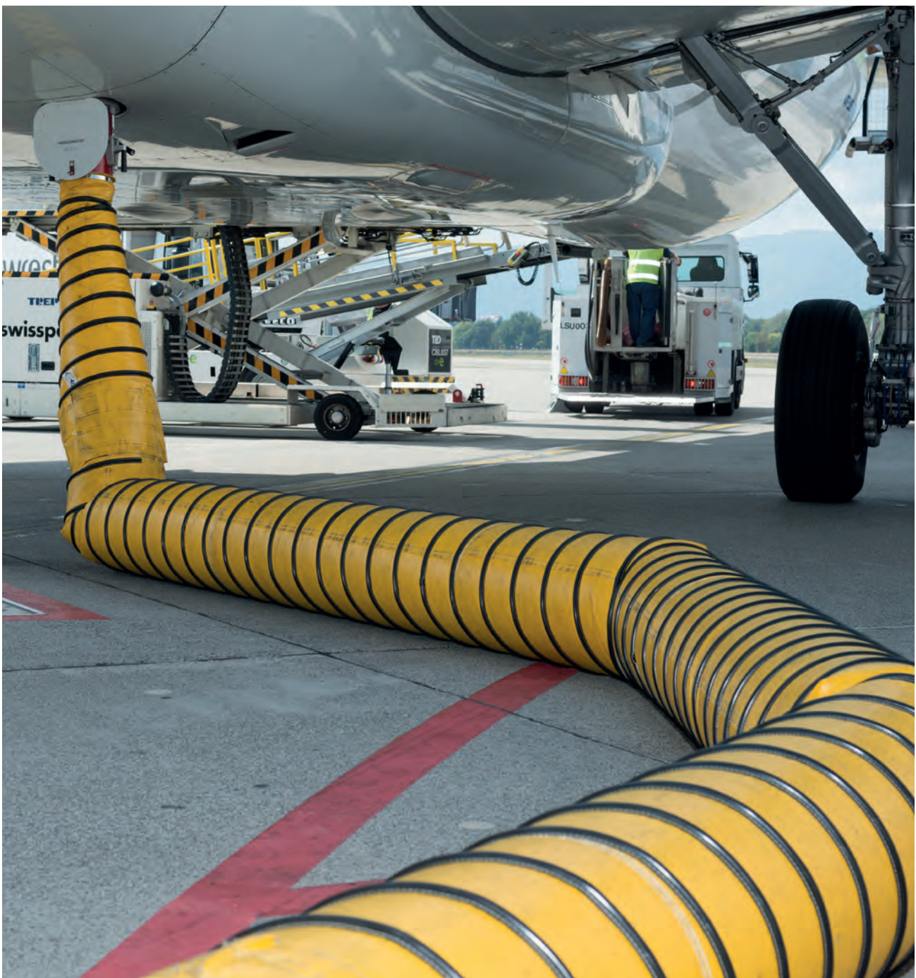
Aircraft air conditioning powered by new heat pumps
